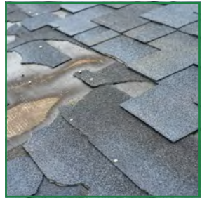
Missing Shingles
